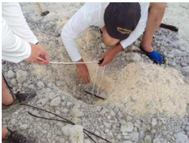
Figure 8 - Luke VK3HJ setting a dead-man (photo K5GS)
